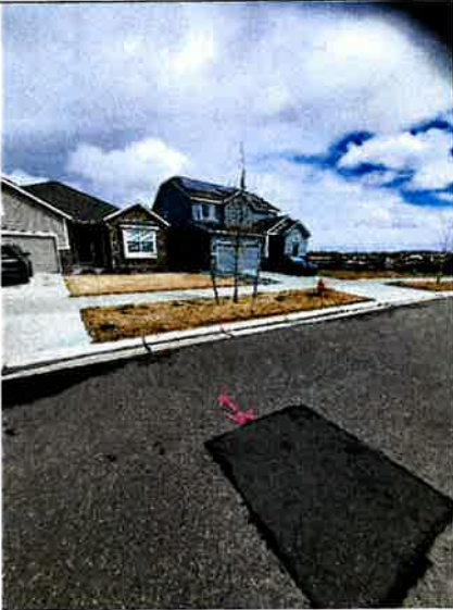
Concrete R&R/Asphalt Patch
