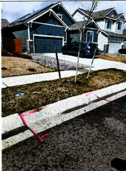
Concrete R&R/Asphalt Patch Back
