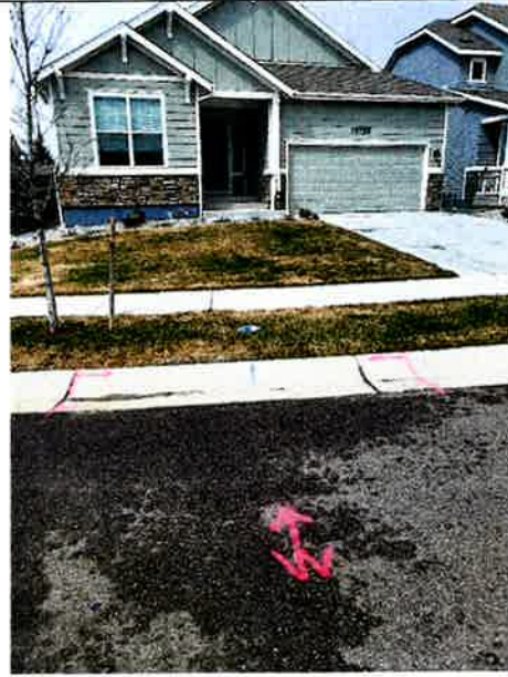
Cut in Water service
