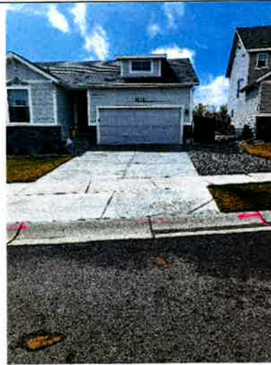
Concrete R&R/Asphalt Patch Back
