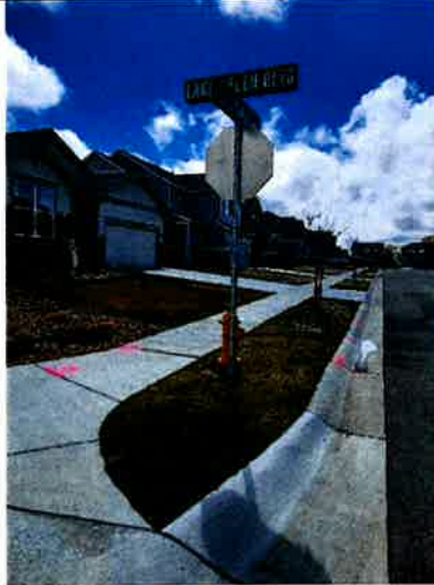
Concrete R&R/Asphalt Patch
