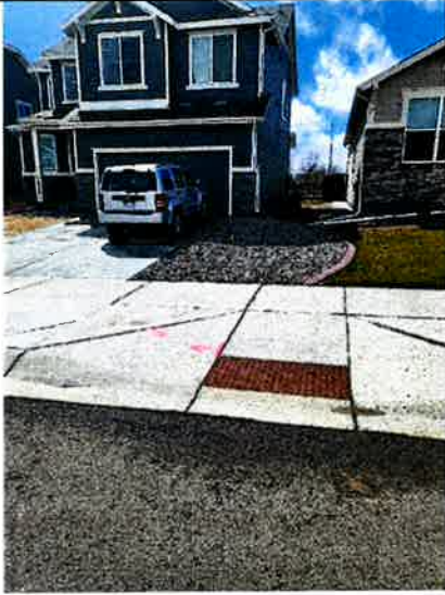
Concrete R&R/Asphalt Patch Back
