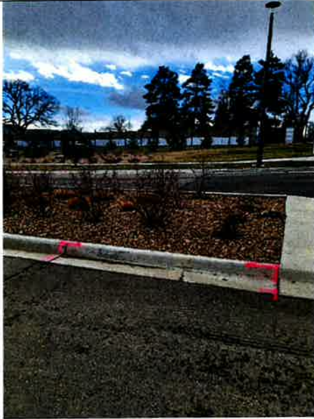
Concrete R&R/Asphalt Patch Back
