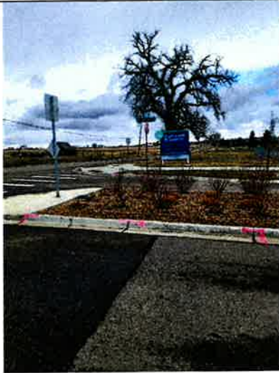
Concrete R&R/Asphalt Patch Back
