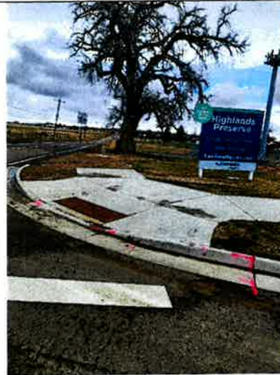
Concrete R&R/Asphalt Patch Back
