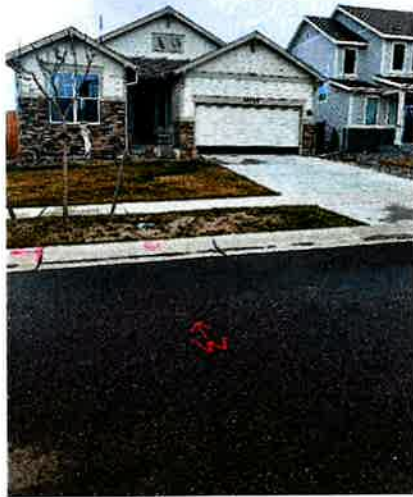
Cut in Water service
