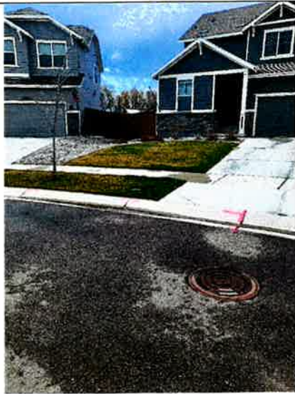
Concrete R&R/Asphalt Patch Back
