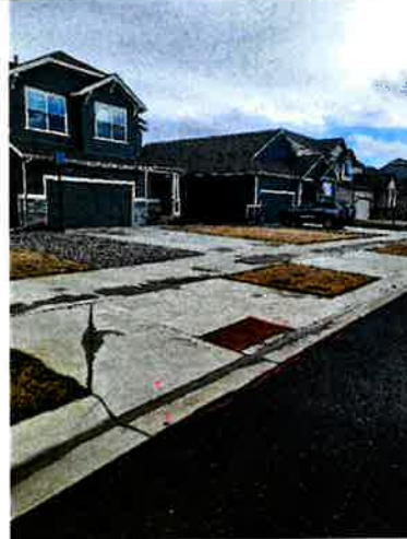
Concrete R&R/Asphalt Patch Back
