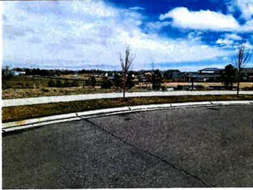
Concrete R&R/Asphalt Patch Back
