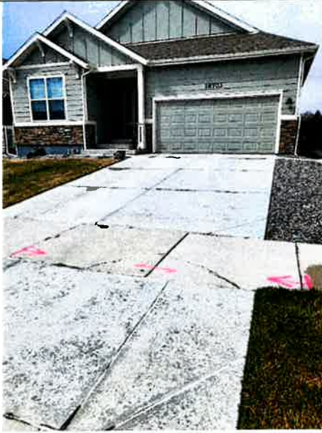
Concrete R&R/Expansion/Seal
