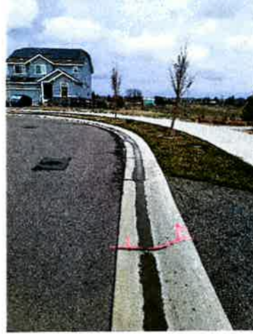
Concrete R&R/Asphalt Patch Back
