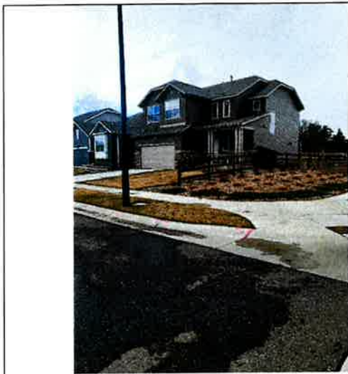
Concrete R&R/Asphalt Patch Back
