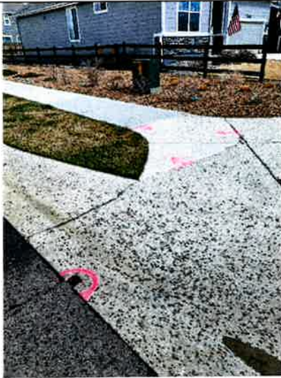
Concrete R&R/Backfill/Sod Patch Concrete
