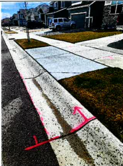
Concrete R&R/Asphalt Patch Back
