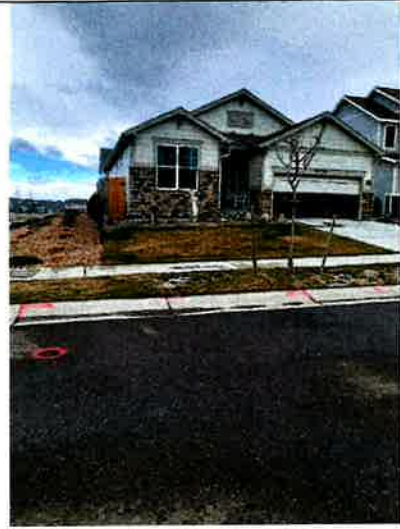
Concrete R&R/Asphalt Patch Back
