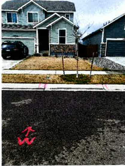
Concrete R&R/Asphalt Patch Back
