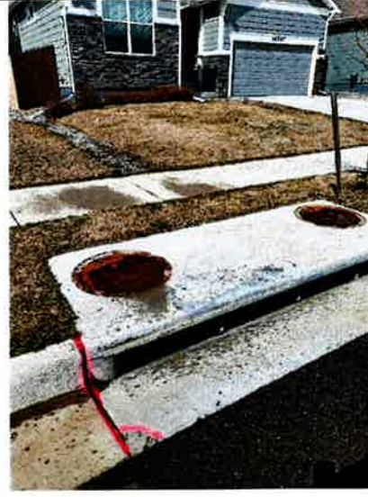
Seal All Expansion/Patch concrete
