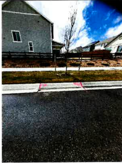
Concrete R&R/Asphalt Patch
