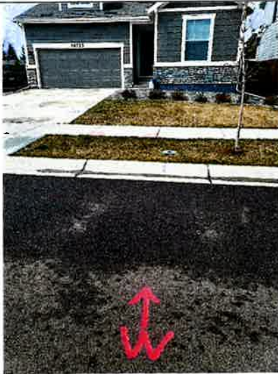
Cut in Water service
