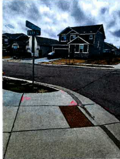
Street Sign meet Town Standards/R&R Concrete
